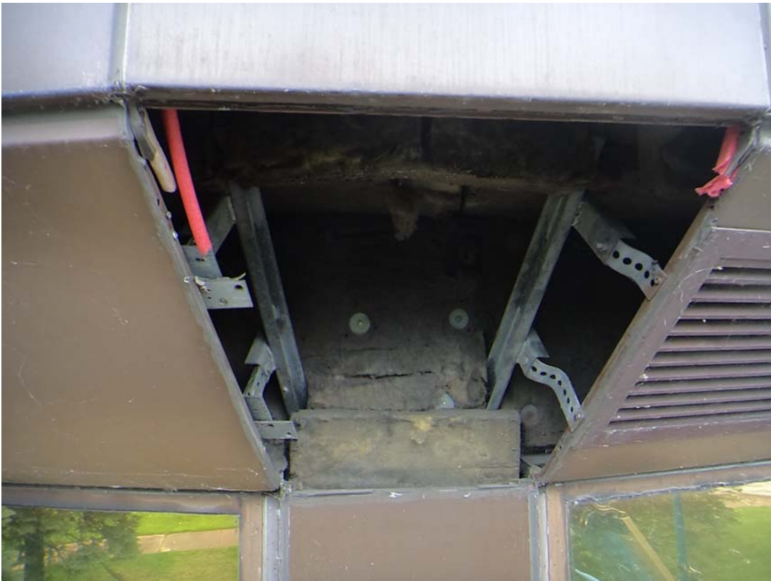
Photo 25 Opening 3 Showing Supports.JPG
