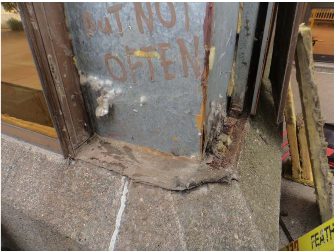
Photo 10 Test Opening on East Elevation.JPG
