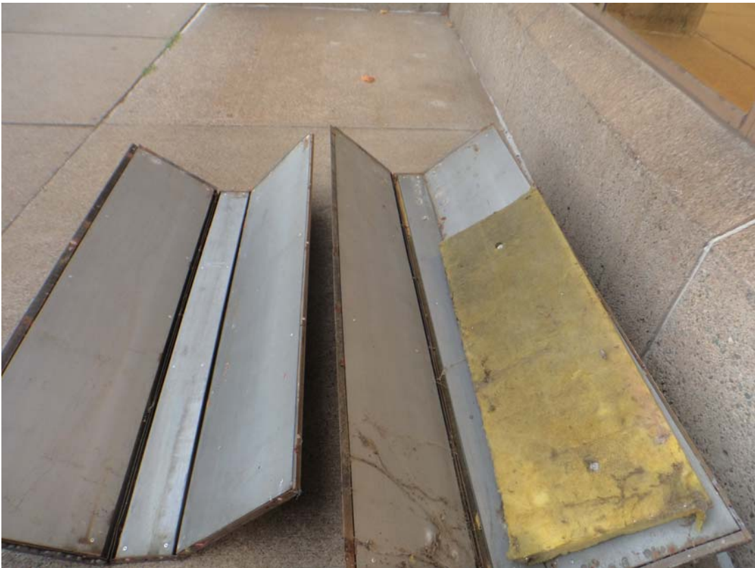
Photo 18 Removed Corner Panels.JPG
