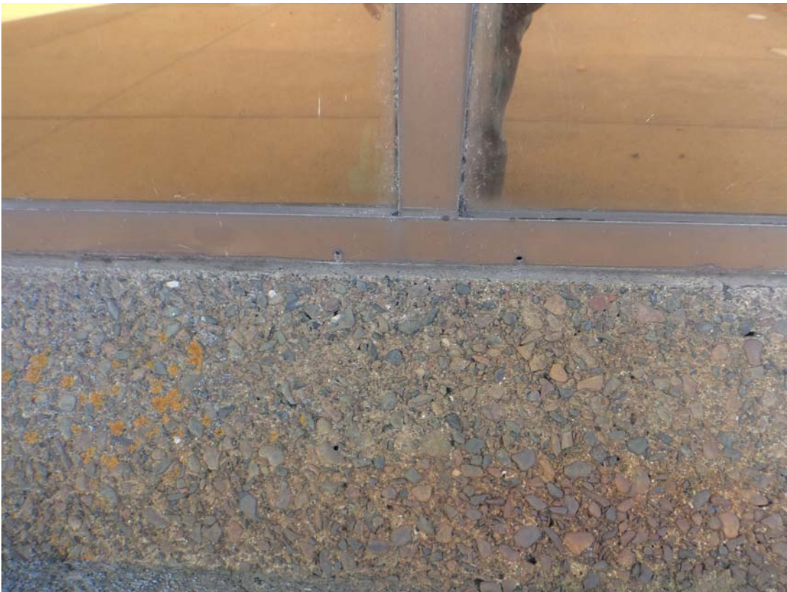
Photo 27 Sill of Window.JPG
