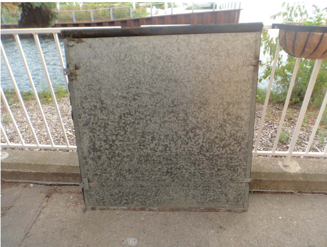
Photo 20 Removed Panel Back.JPG
