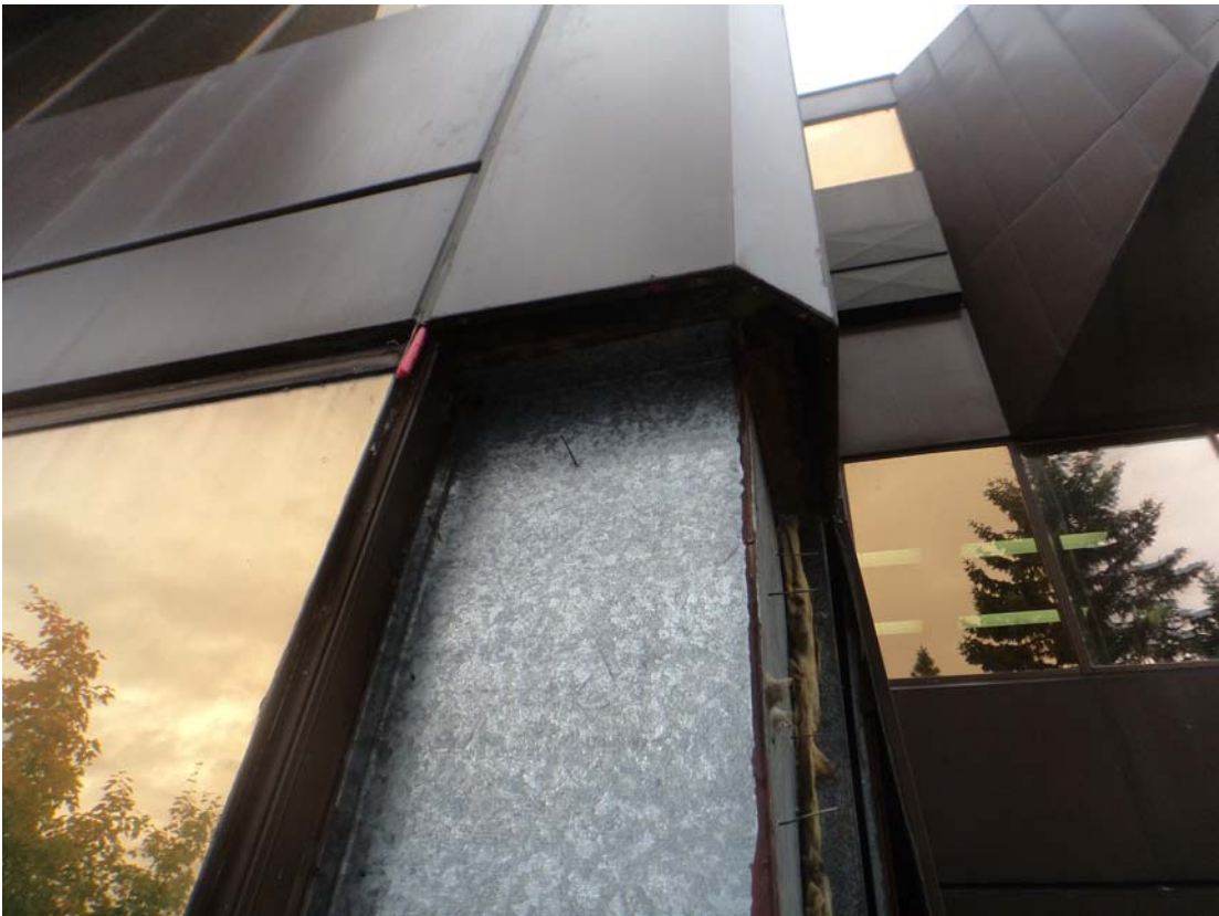
Photo 9 Test Opening on East Elvation.JPG
